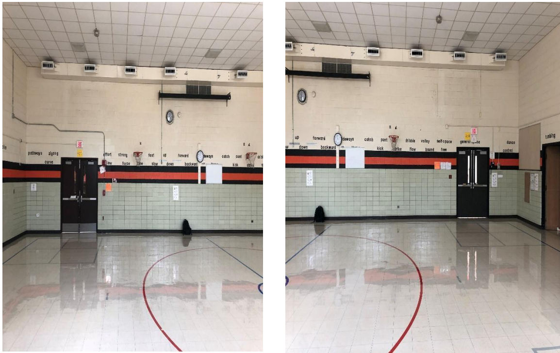
Figure 2. Side-by-side photo composition showing the gymnasium's west wall. 5
