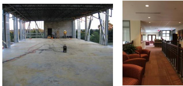
Figure 3. VUAC during and after construction conditions
