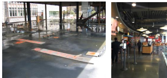
Figure 1. ASAB during and after construction condition
