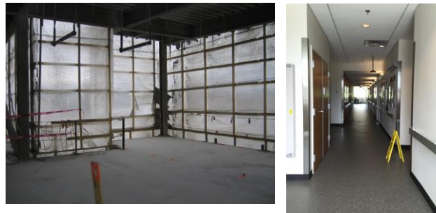
Figure 2. IDRF during and after construction conditions
