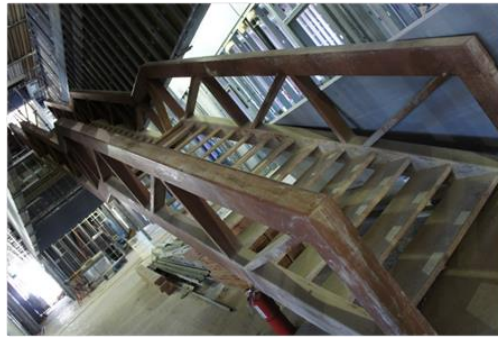
Figure 9. photo of VT Classroom staircase
