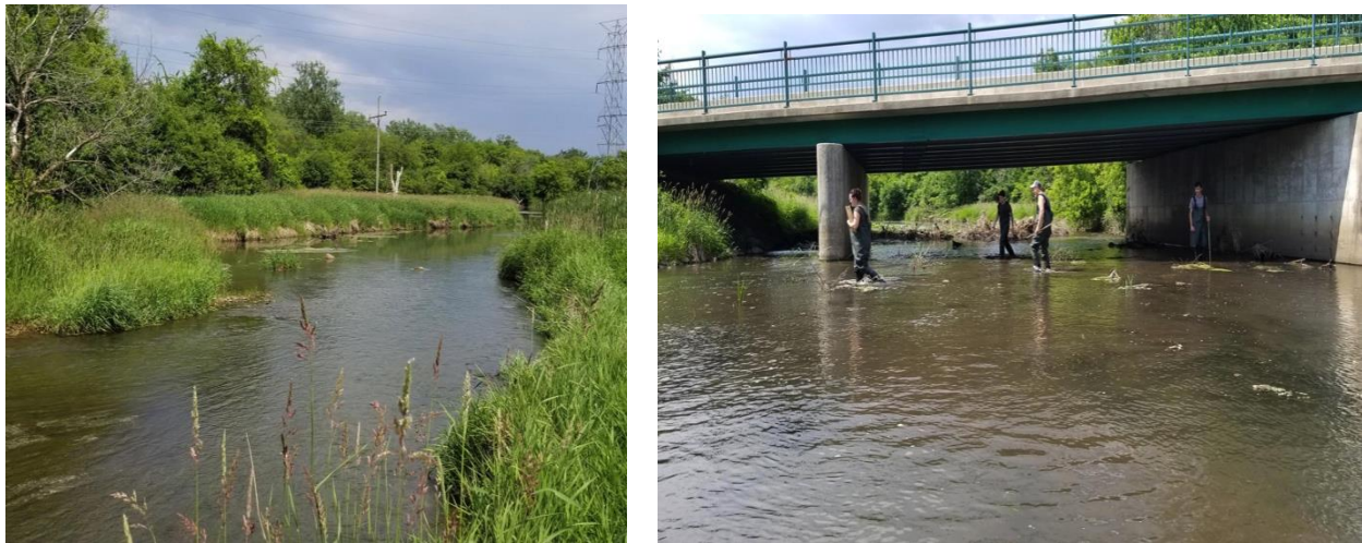
Figure 2. Lily Cache Creek at Four Seasons Baseball Fields, Plainfield, IL. a. Established Reach with no man-made structure (Left), b. Adjacent Downstream reach with vehicle overpass (Right)
